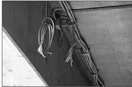
X-ECH for fastening bunched cables
