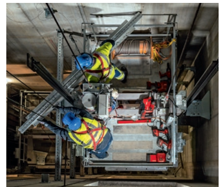
Lightweight beam can be moved by single person
