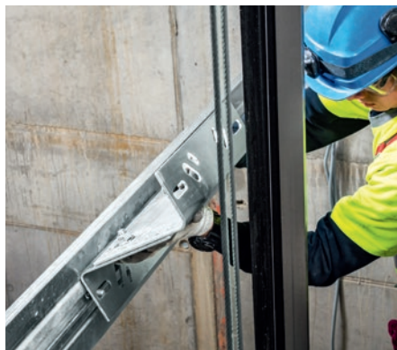
Attach rail connector with T-bolt in C-channel
