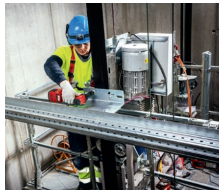
Lock bolts after final adjustments
