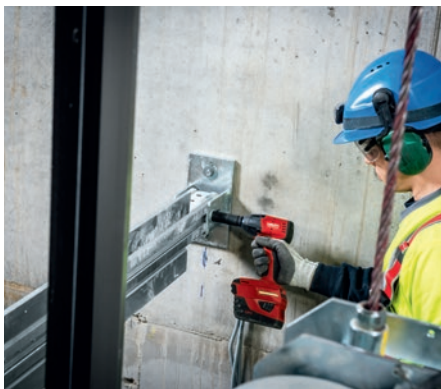
Locking bolts in slots after final adjustment
