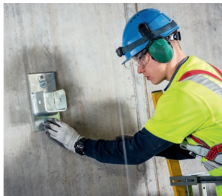
U-connectors safely hold beams without fasteners
